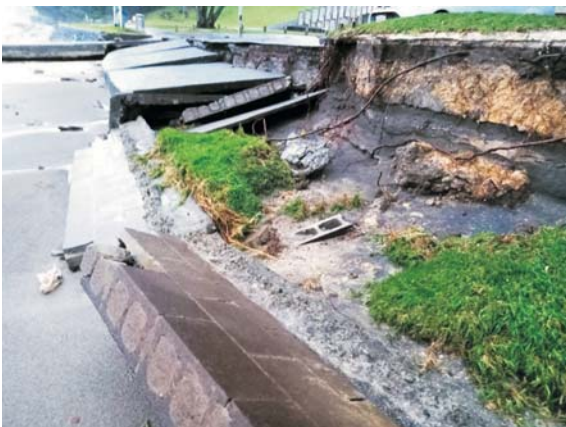
Figure 9: Seawall failure, post Cyclone Gabrielle Storm.
