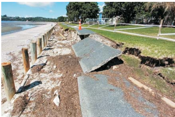
Figure 15: Failed timber seawall, post Cyclone Gabrielle.
