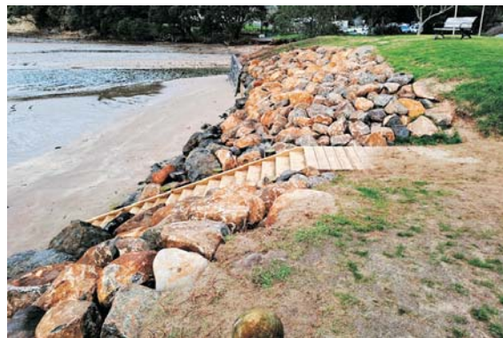
Figure 13: Renewed rock armouring and access stair.
