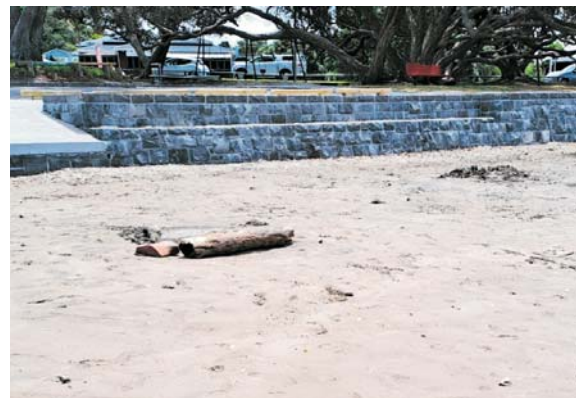
Figure 10: Renewed masonry seawall and stepping detail at Murrays Bay.
