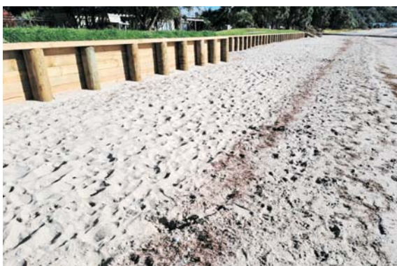
Figure 16: Renewed timber seawall set landward, and adjacent dry high tide beach.
