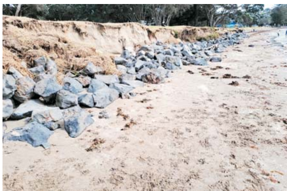
Figure 11: Exposed backstop rock armouring on Browns Bay beach, to become naturalised dune section, post ex Cyclone Lola Storm.
