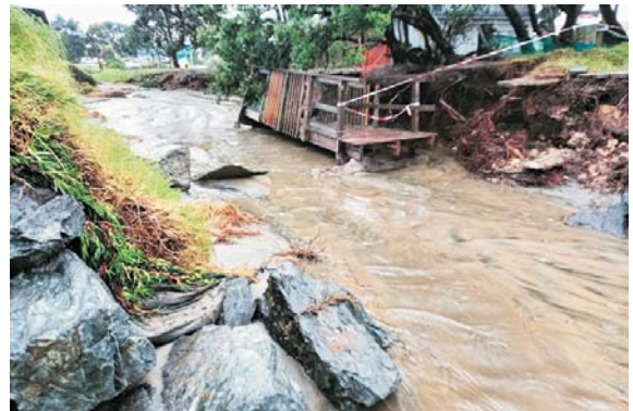
Figure 7: Post Gabrielle storm, footbridge failure.
