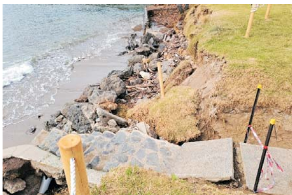
Figure 12: The southern end of Browns Bay, with reserve erosion, exposed backstop armouring, and failed steps, post ex Cyclone Lola.
