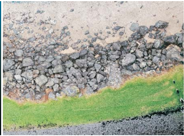
Point cloud generated from UAV survey conducted in 2022
