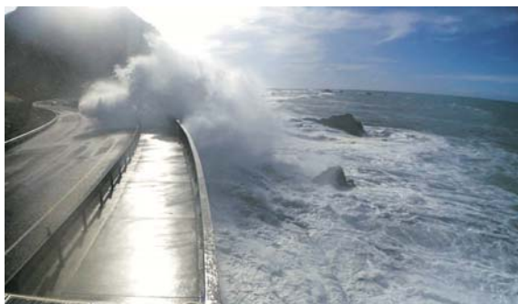
Figure 1: Monitoring imagery of wave overtopping at Ohau Point, north of Kaikōura (Source: Shand et al., 2021).
