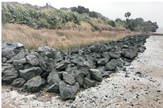
Figure 4: Example of a hybrid coastal defence solution at Wattle Downs, Auckland (Photo: Tonkin+Taylor).
