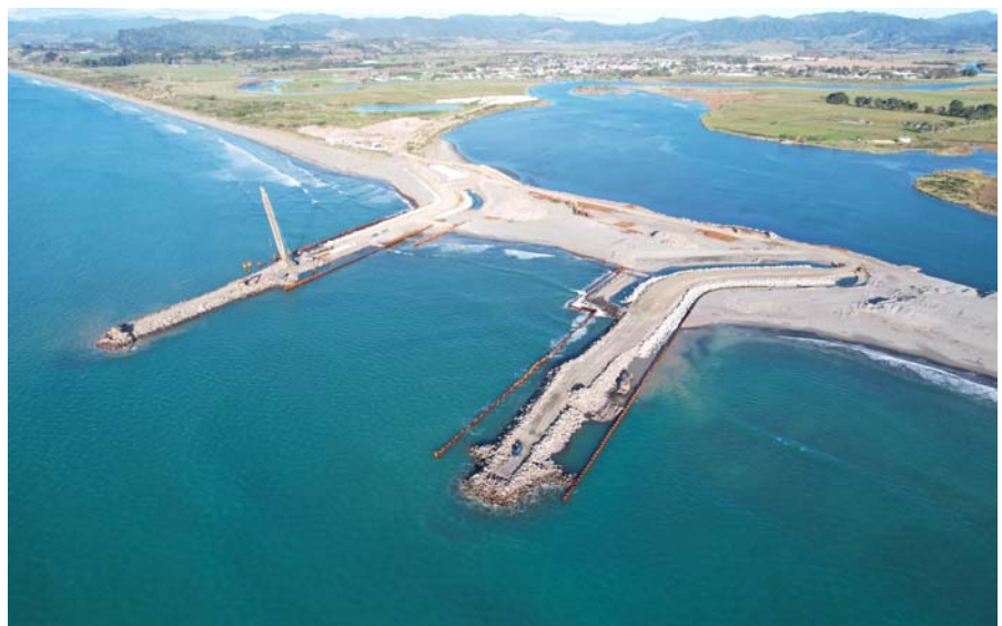
Ōpōtiki Harbour development (Photo: HEB Construction).
