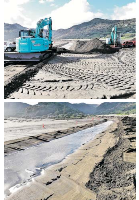
Stream realignment works, June 2020 (Photo: Matthew McNeil).
