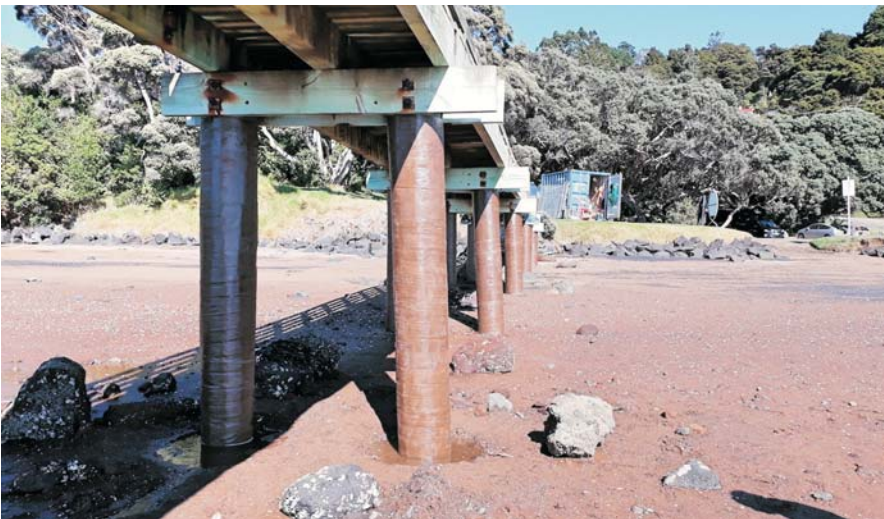
Top, Cornwallis Wharf; Bottom, Denso pile wrapping (Photos: Christoph Soltau).
