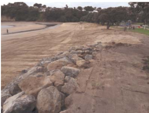
Removal of relic rock armour and reprofiling of coastal edge (Photo: Natasha Carpenter, Principal Coastal Specialist, AC).
