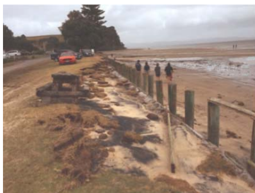
Damage to vertical timber seawall at Logan Drive (Photo: Jo Morriss, Coastal Scientist, AC).
