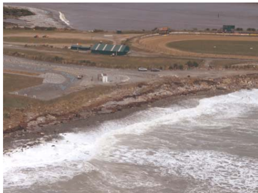
Erosion along the front of the old Cobden Dump site with the Grey River in the background (Photo: West Coast Regional Council).
