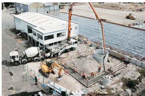
Constructing the new wastewater treatment plant, which services the entire hard stand area (Photo: Vessel Works).
