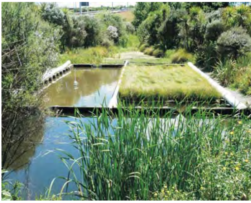
The stormwater pond after the floating vegetated island had been in place for one year. Photo: University of Auckland.
