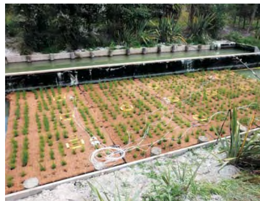
The floating vegetated island the day it was installed (Dec 2010).
