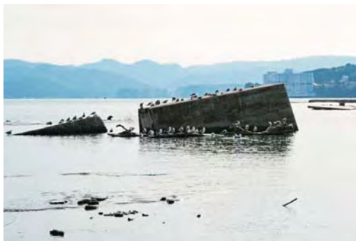
Figure 3: Failed breakwater in the harbour of Minami-Sanriku City (Dec. 2011). Photo: C Gomez.
