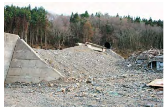
Figure 5: Former train track and bridge between Rikuzentakata and Minami-Sanriku, destroyed by the tsunami. To the right: debris deposits have filled low-lying areas in front of the raised train line, with only the tips of remaining structures now visible (Dec. 2011). Photo: C Gomez.
