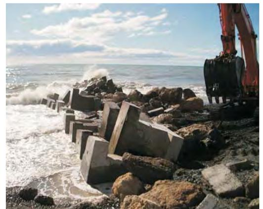
*Figure 5: Maintenance work to the Haumoana groyne with 8-tonne blocks*
