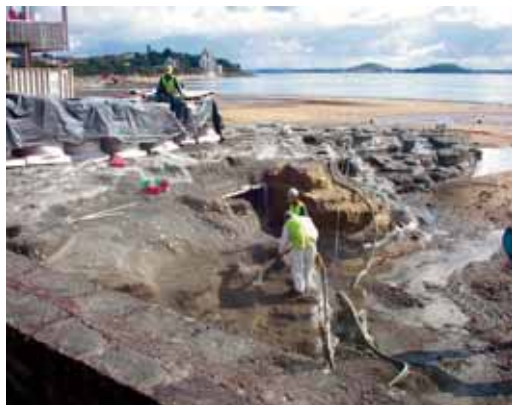
Naturalistic headlands were created at either end of Kohimarama Beach using 'sandcrete'. Photo by Patrick Reynolds.
