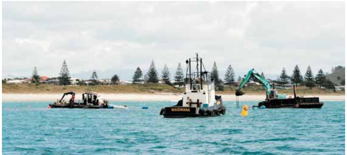
Very flat seas are required to pump sand into the giant bags that make up the Mount Reef (Photo: Dean Tully)
