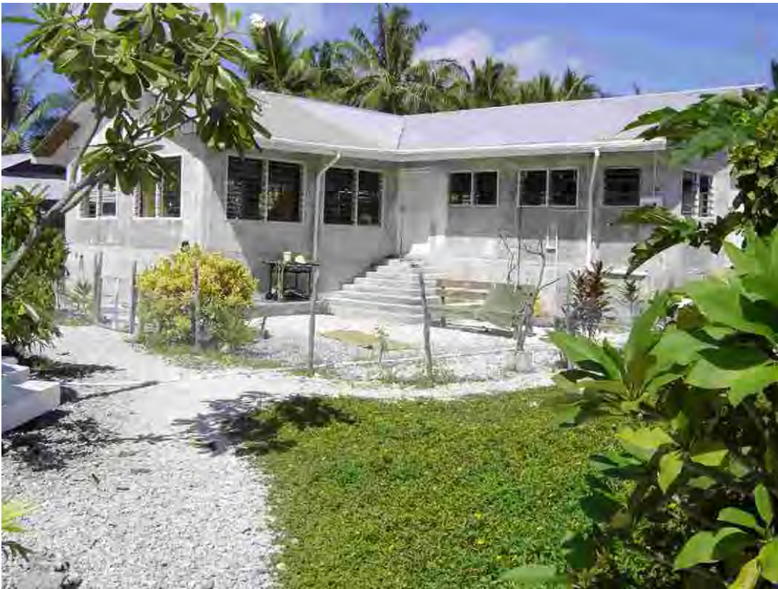
Figure 3: A typical house built with Tokelau Government housing grant assistance. The water tank raises the floor level about 1 m above the ground level reducing the risk of inundation. (NIWA)
