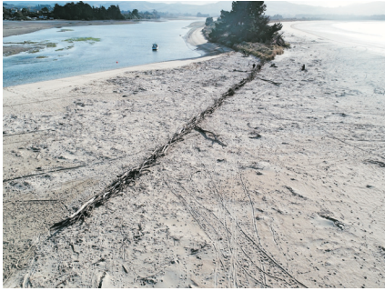
Aerial view of the driftwood windbreak on the day of construction. Fence alignment was determined based on the local wind conditions and took into consideration the way that the sand spit has accreted in the past (Photo: Tom Simons-Smith).
