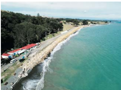
Aerial view of Clifton revetment (Photo: Hastings District Council).
