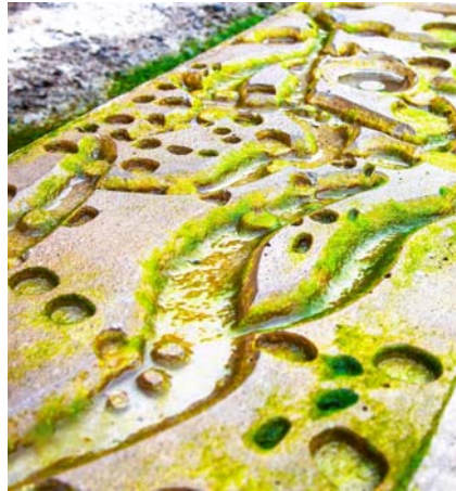
Artificial rock pools (left) and textured sea walls (right) recently installed as part of coastal development in Wellington Harbour (Photos: Annie Graham, GWRC, left; Shelley McMurtrie, EOS Ecology, right).
