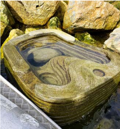
Artificial rock pools (left) and textured sea walls (right) recently installed as part of coastal development in Wellington Harbour (Photos: Annie Graham, GWRC, left; Shelley McMurtrie, EOS Ecology, right).
