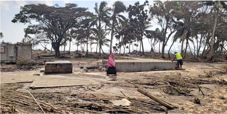
Figure 2: Tsunami damage in Ha'atafu (Photo: Moana Paea, Ha'atafu Beach Resort).
