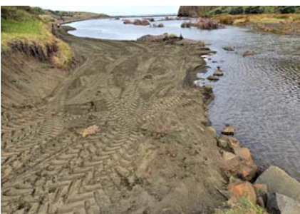
Figure 5: Reinstated vehicle accessway, 6 October 2021.
