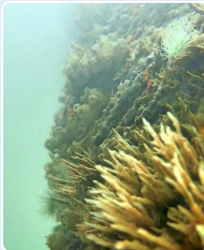
Pile jackets ©ECONcrete.
