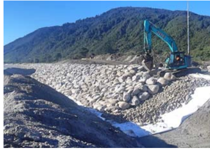
Seawall construction showing geofabric and rock layering (Photo: Paulette Birchfield).
