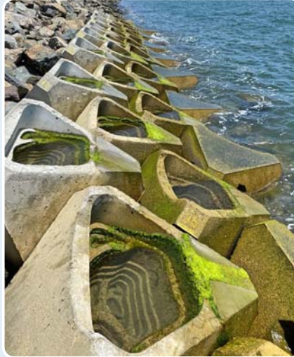
Coastal lock units ©ECONcrete.
