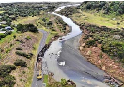
Figure 2: Bethells Road flood damage under repair.
