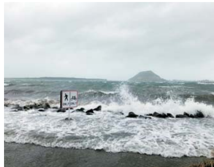
Figure 2: Wave overtopping near Kulim Park, Tauranga.
