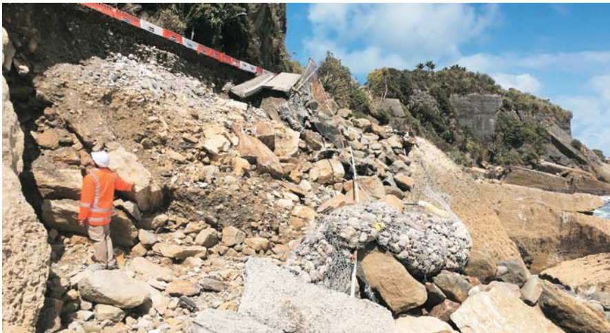
Figure 4: Punakaiki section (SH6) damaged after ex-tropical cyclone Fehi (Photo: WSP Opus).
