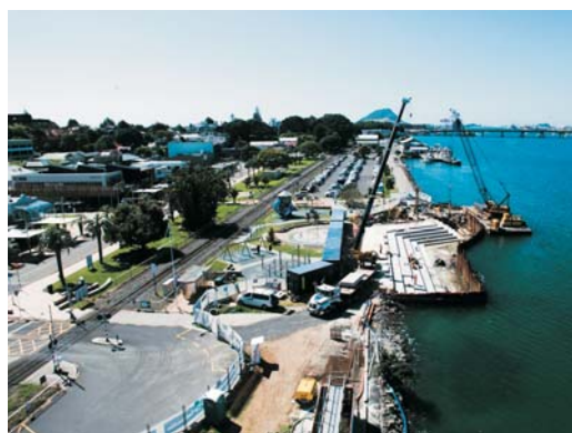
Cranes move the precast concrete steps into place (Photo: HEB Construction).
