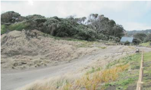
Figure 3: Completion of stage 1 with realignment of car park and dune regrading.
