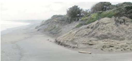
Figure 4: View of proposed stage 2 works outlining the over-steepened dunes.
