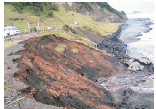
Figure 2: Coastal erosion at the southern car park, 2006.
