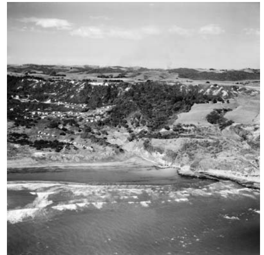
Figure 1: Historical photo of Muriwai beach, 2 April 1957 depicting what was a natural valley feature prior to infilling and reclamation.
