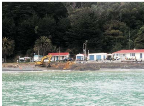
During seawall construction.
