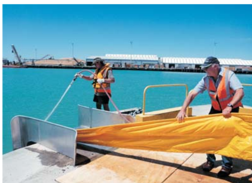
Use of boom protector over the edge of the wharf during deployment and recovery of the boom.
