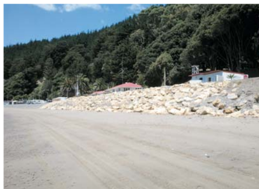
After seawall completion.
