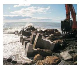
Figure 5: Maintenance work to the Haumoana groyne with 8-tonne blocks
