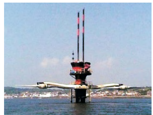
Figure 2: Seagen – in raised position to show tidal turbines
