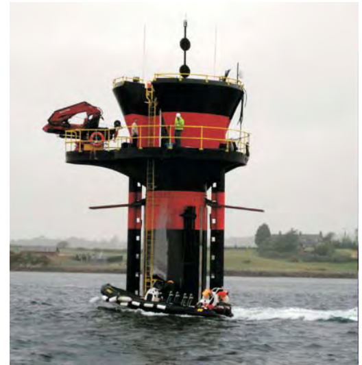
Figure 1: Seagen tidal turbine in Strangford Loch, Northern Ireland
