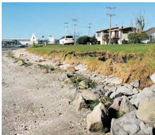
Inner harbour erosion (left) causing risk to public amenity and infrastructure. Subsequent beach enhancement (right) after beach re-nourishment and control structure.
