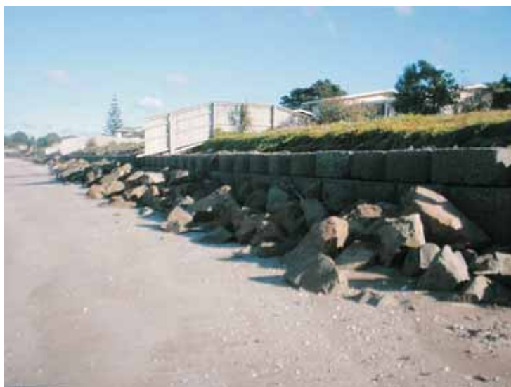
Photo 1: Seawall at Buffalo Beach, Whitianga. (Photo courtesy of Beca.)
