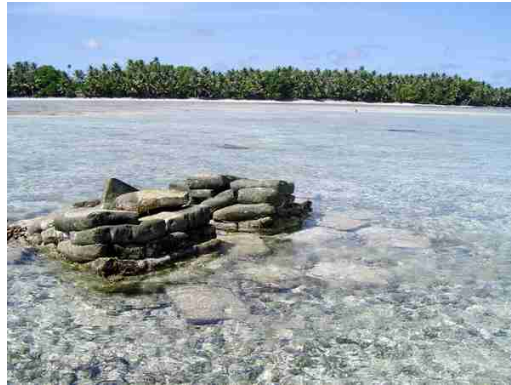
Figure 3: Bags of concrete stranded on the reef flat of Nukulaelae after a tender boat capsized crossing the reef. (NIWA)
