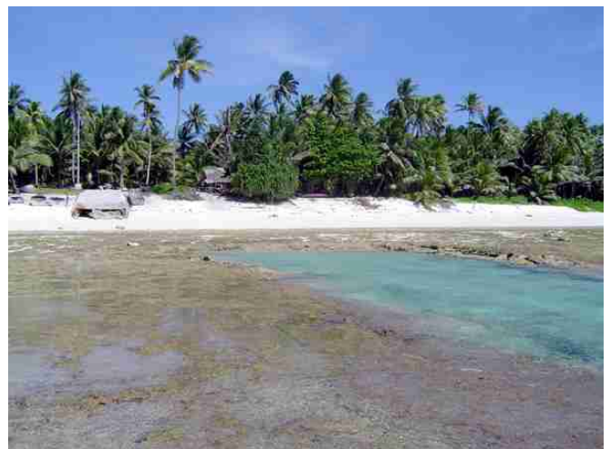
Figure 4: The reef channel on Niutao atoll. Note the erosion being caused by the concrete ramp, part of which has been removed. (NIWA)
