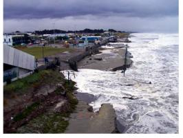
Figure 1: Erosion of sand fences, New Brighton Beach
